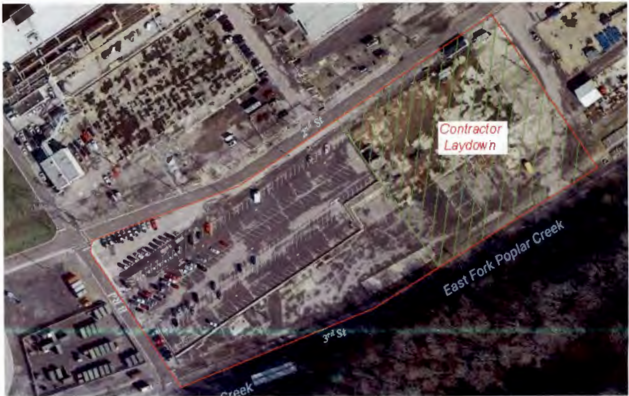
TREATMENT PLANT SITE
